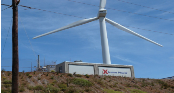
Xtreme Power KWP 1
